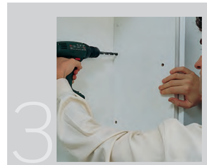
3 Drill the 8 holes needed to fit the plate-rack onto the points marked out with the punch tool.
